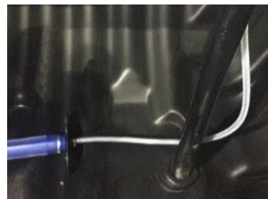
Place Diffuser Onto The Centre Of The Tank Floor
