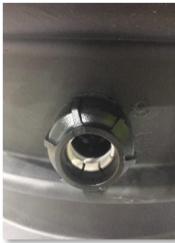
Cut hole in manway to position pump outlet pipe
